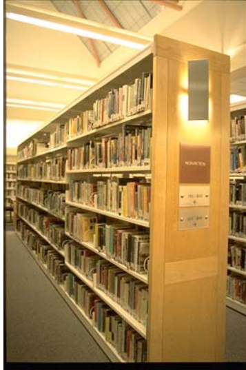
Illustration 6: Direct-indirect lighting runs perpendicular to the stacks at the Albany Public Library, and the lighting is very even across the entire stack face.
