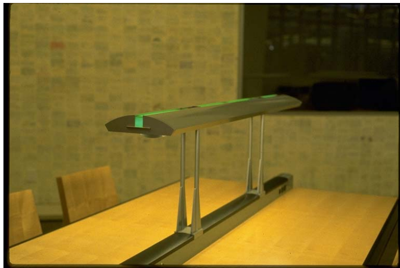
Illustration 9: Table lamps must light the table evenly and be very sturdy. The base of these lamps at the San Francisco Main Library also includes power and data wiring.
