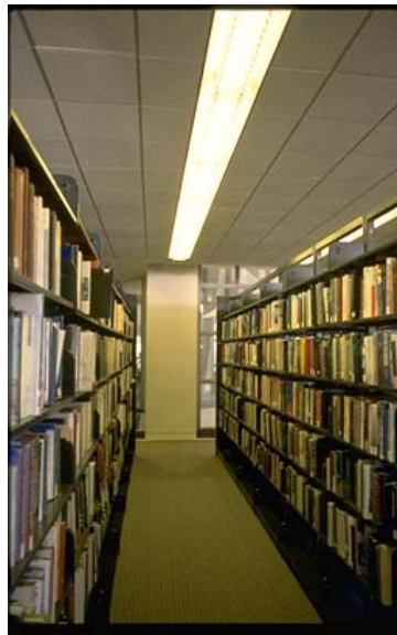
Illustration 4: Stack lighting runs parallel to the stacks at the San Francisco Main Library, and the lighting is very even from top to bottom of each stack.
