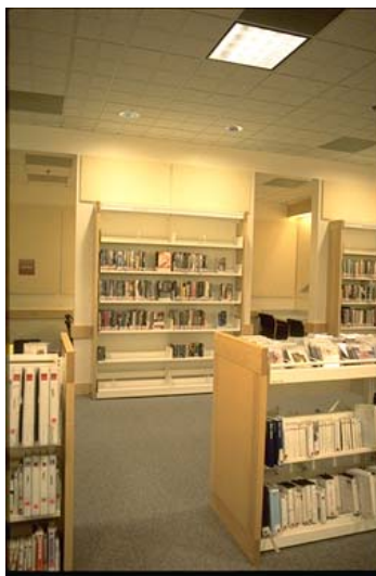
Illustration 11: With additional wall washers, the perimeter bookshelves are lit and the space feels brighter, even though the average lighting level on the tables is the same as in Illustration 10.
