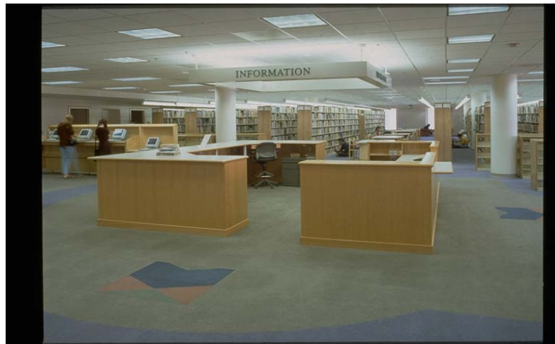
Illustration 8: Recessed fixtures with parabolic louvers provide low-glare lighting at the Sacramento Central Library.
