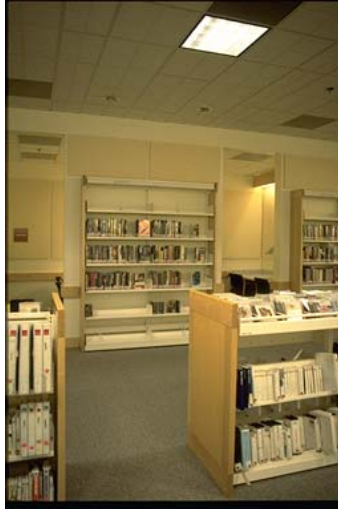
Illustration 10: Although recessed 2'x2' fixtures with parabolic louvers can provide low-glare lighting for reading tables, they do not light the perimeter of the space very well.
